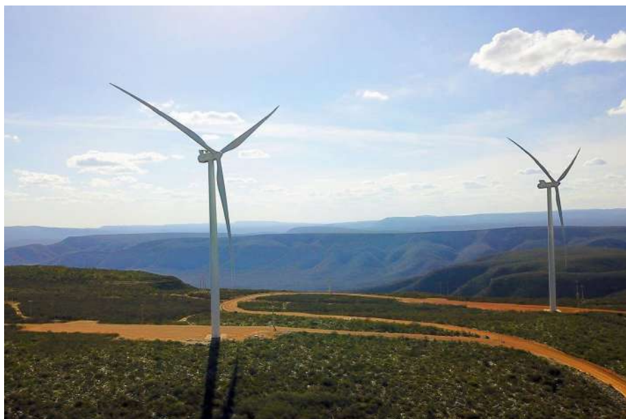
ENEL GREEN POWER
